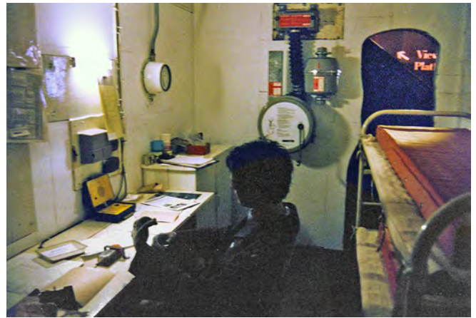
The recreated post at the Museum of Lancashire in 1994 – the hole which Tony created through the 'concrete' wall can be seen to the right, as can the sign to the viewing platform. The Luwa air system is in the centre of the picture, its filter in the bypassed, i.e. the normal position. The post office termination and test box are in front of the observer along with new style teletalk. The later type of FSM meter is shown buried in the desk, with a strap over it to prevent theft! Photo Mike Norris
